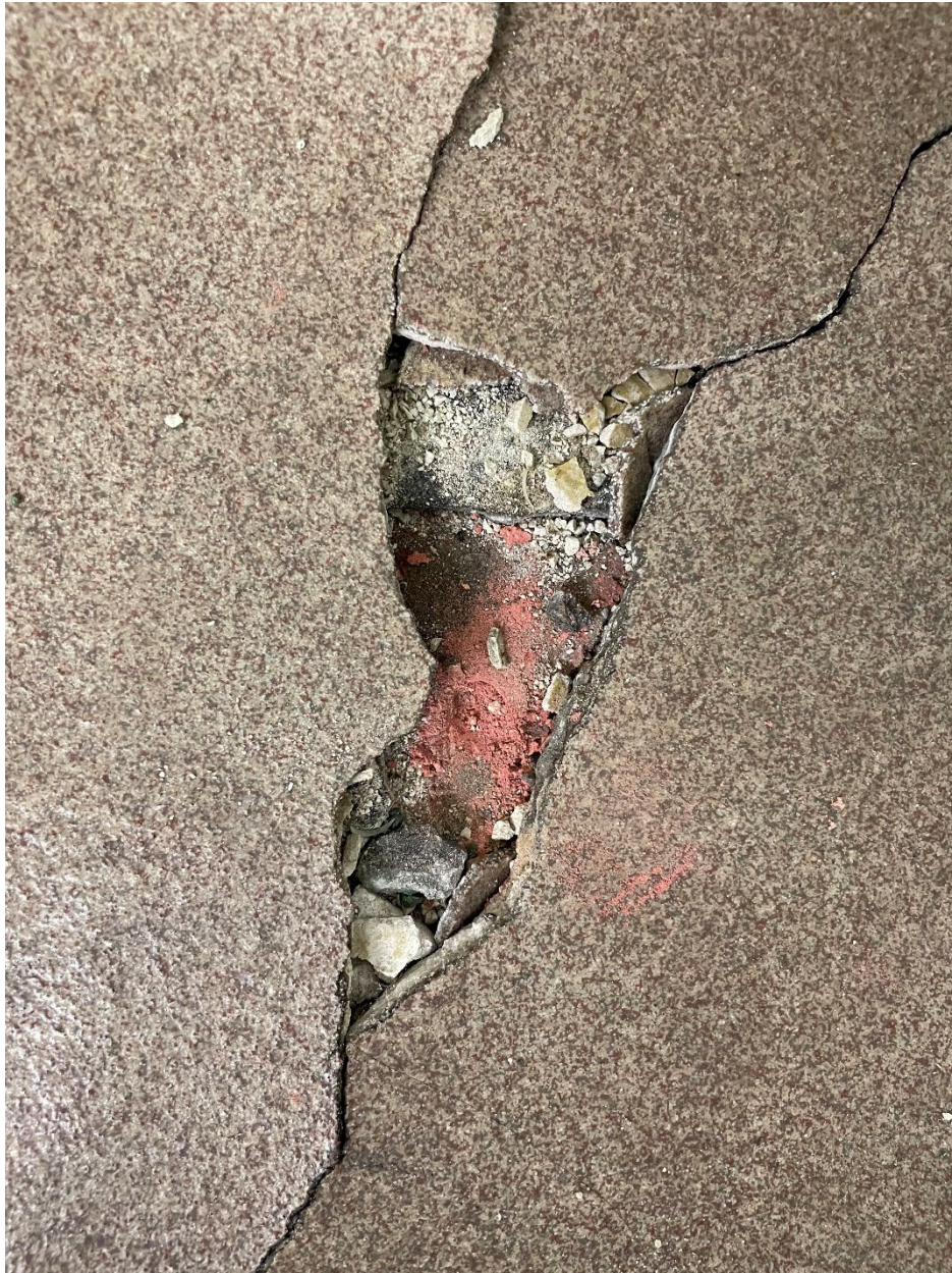
Photo 1 – Concrete Leveler – Pink (ACM) Restroom W203
