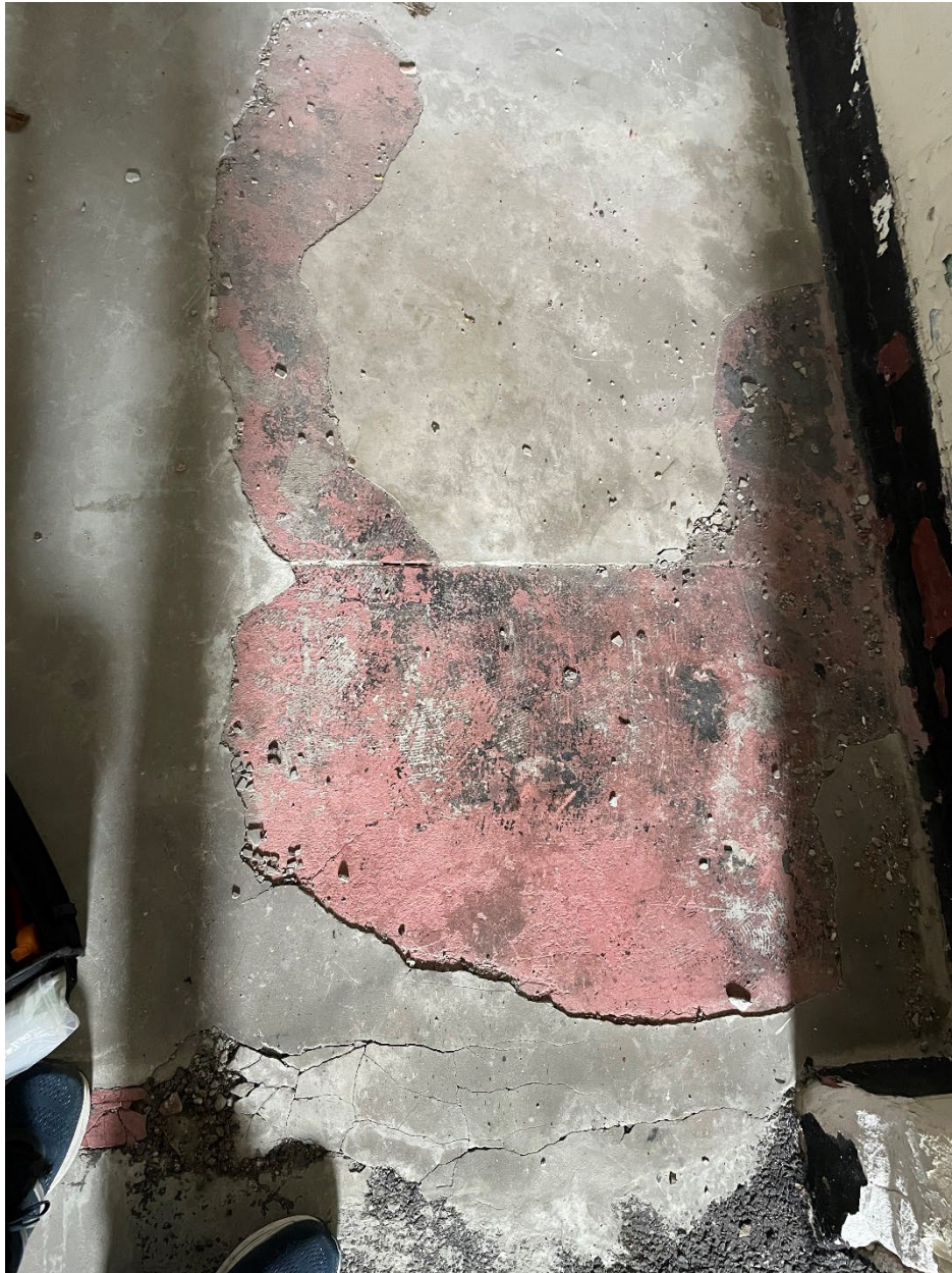
Photo 3 - Concrete Leveler – Pink and Black Mastic (ACM) SW Men's Bathroom
