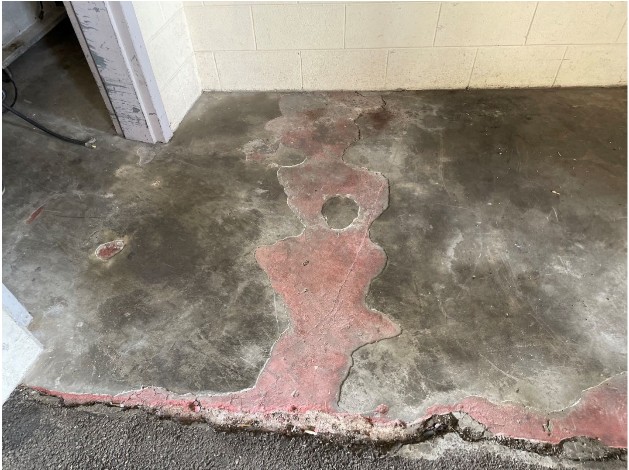
Photo 2 – Concrete Leveler – Pink (ACM) SW Men's Bathroom
